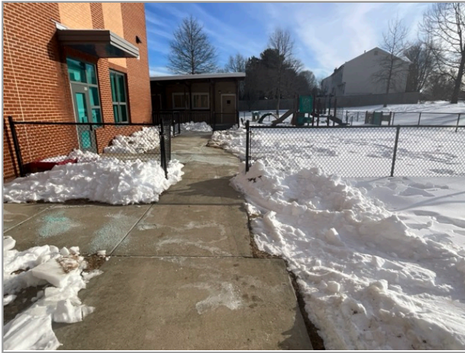
ACCESSIBLE ROUTE TO PLAYGROUND
