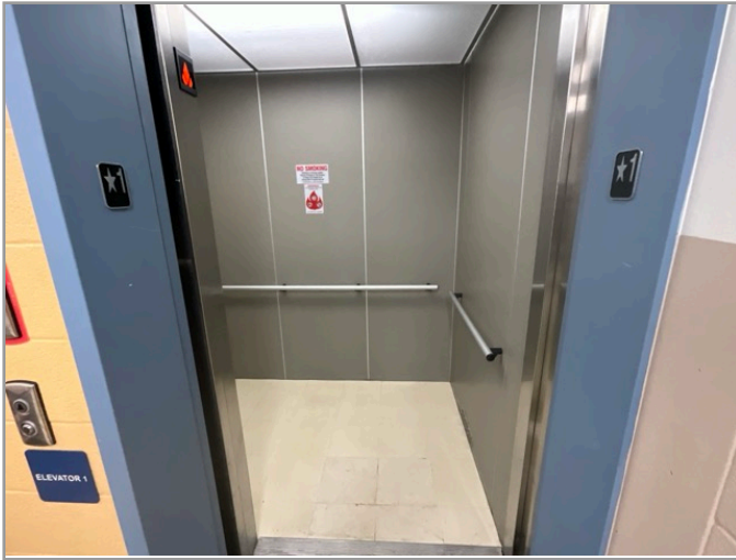
LOBBY LOOKING AT CABS
