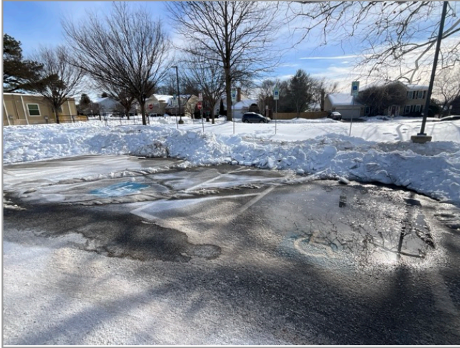
OVERVIEW OF ACCESSIBLE PARKING AREA
