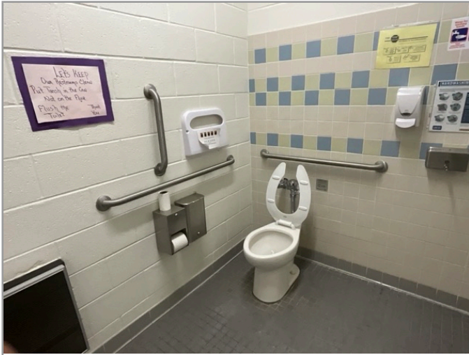
TOILET STALL OVERVIEW
